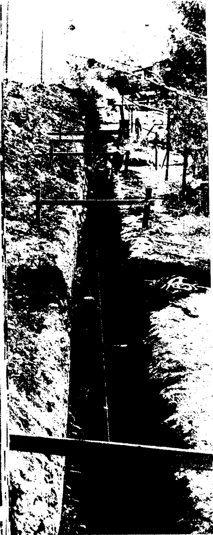
J. Floyd Edmonds, Henry C. Spraker and Robert E. Stoots laying a new sewer line in town.
