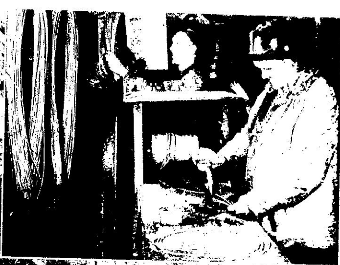
Roy L. Lawson and Robert Whitt preparing blasting fuse at the underground powder station.
