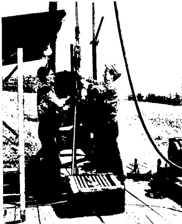
Marvin Dean and Roby Stoots lowering drill rods in a diamond drill hole.
