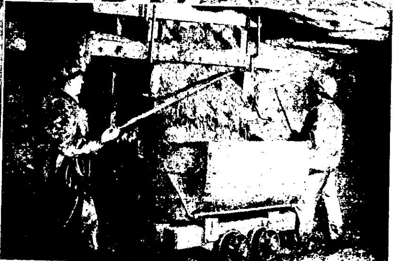
Ransom A. Alley and Lee V. Alley loading ore from a stope chute.
