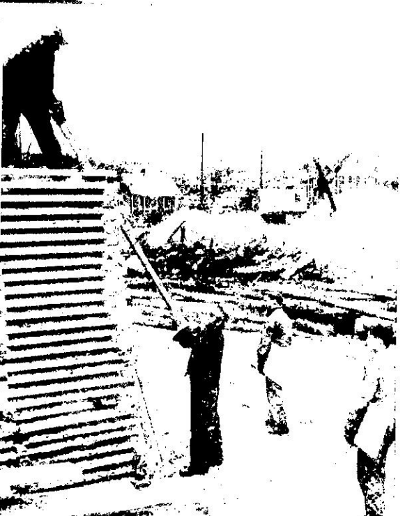
Chester W. Arnold, Jr., Robert G. Sisk, C. Paul Dunford and James J. Harmon stacking green lumber in racks for air drying.
